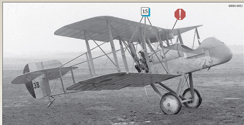
AMC DH.2 5938 displays its factory fresh finish of translucent clear doped Irish Linen with grey painted wood and metal parts. Note the position of the emergency gravity petrol tank under the port top wing. This is almost certainly how 5964 would have appeared when it was initially delivered to 24 Squadron on 2 April 1916. By the time 5964 was being flown by Lanoe Hawker in November 1916 it would have undergone quite a few changes including the addition of a 4 blade propeller, relocating the emergency petrol tank to the top of the wing and having the upper surfaces overpainted with PC10.
